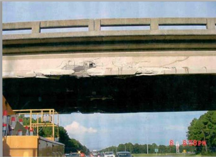
Figure 227—Girder damage from vehicle impact in July of 2001
