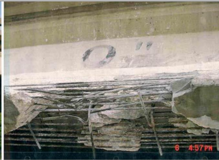
Figure 227—Girder damage from vehicle impact in July of 2001
